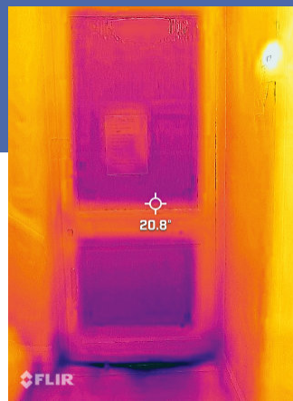
This bathroom always seems cold. The IR camera shows why: it was built into a roof but no insulation was added. A builder could add insulation from outside (by temporarily removing tiles) and make it much warmer.
