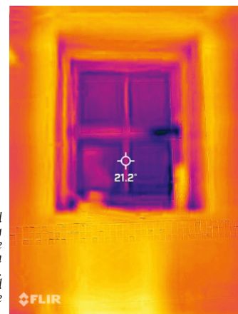
In this image from outside a HGS home, the lower window is single-glazed and is clearly losing more heat than the window above that has secondary glazing – more proof that secondary glazing is highly effective.
